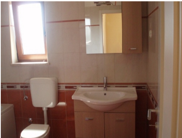
One of the two bathrooms
